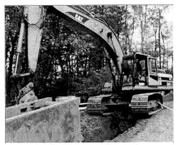
The track-hoe involved in this incident was pulling a trench shield forward in a trench for a sewer system when a hook failed and the rigging snapped loose.
