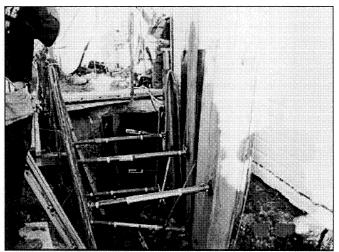
Figure 3. Shoring installation
