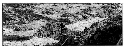
Photo 1. Illustrates the usual depth of the footings and the gravel fill. Photo courtesy of NCOSHA.
